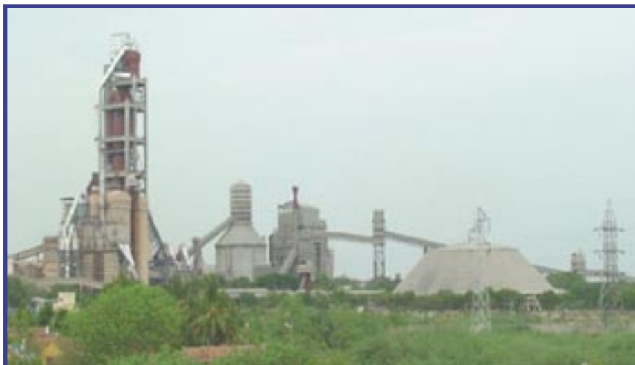
Figure 7: Overview of the DCBL plant at Dalmiapuram, India.
