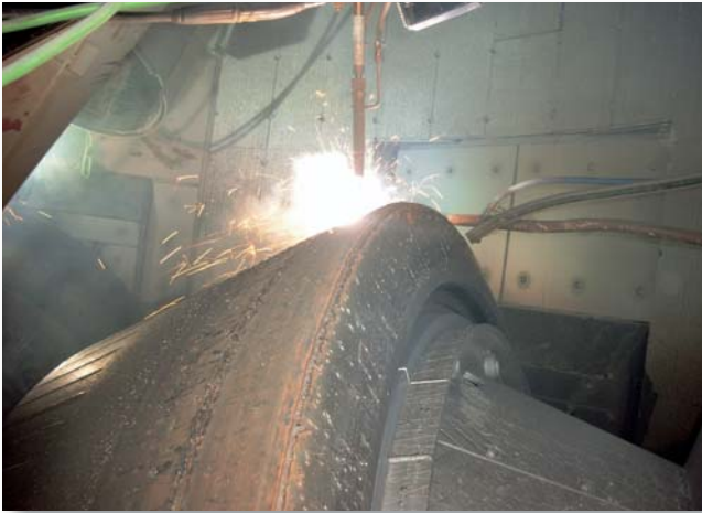
Figure 6: In-situ hard-facing of the roller surfaces
