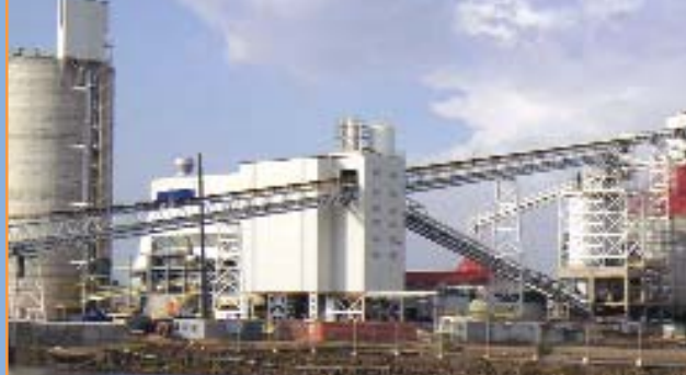
Figure 8. LM 56.2+2 in Thi Vai plant of Holcim Vietnam.
